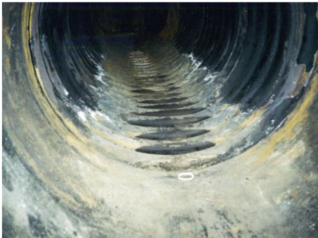
Fig. 4 Deposit in fire chamber after the combustion of 2000 t animal fat
